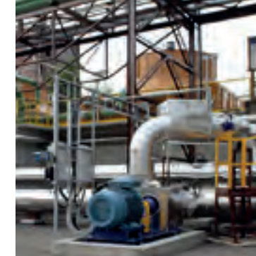
Desulphurisation of the Coke Plant
