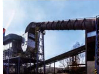
De-dusting of cooling belts, Sinter Plant, northern part
