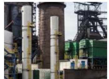
Blast Furnace 3 - charging system de-dusting
