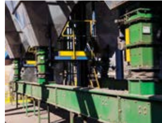
De-dusting of cooling belts, Sinter Plant, southern part
