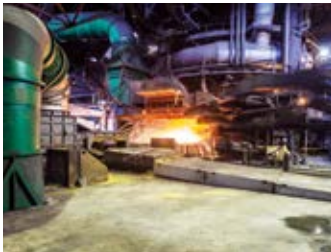
Blast Furnace 2 - cast house de-dusting
